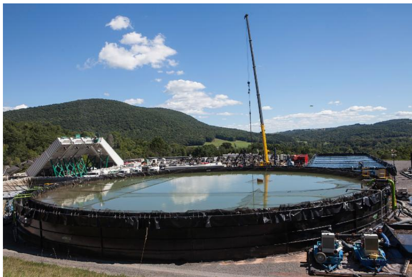
An open-air container at the Yeagle Road well holds flowback (frack) water that will be treated and re-used until it is finally hauled to a toxic waste injection disposal site. (Note the netting required to prevent birds from landing in the tank is largely under water.)
